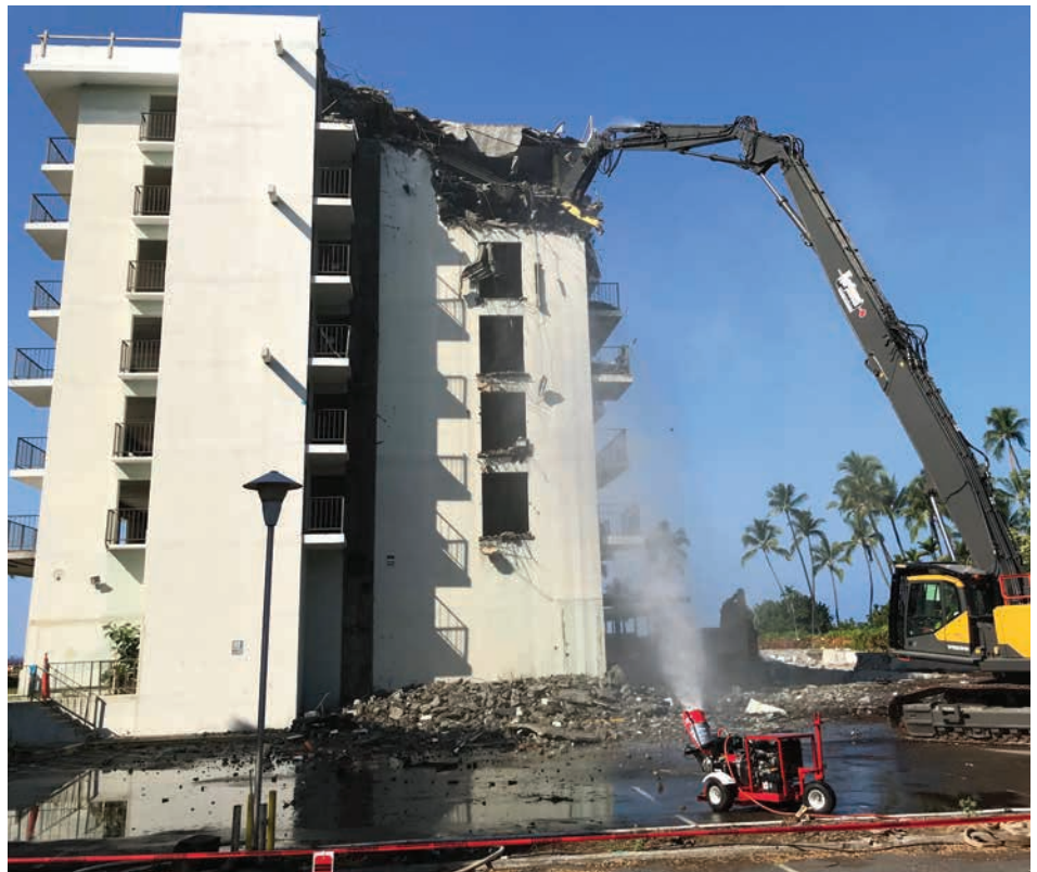
High reach structure removal. Photo provided by Kiewit Building Group, Inc.
