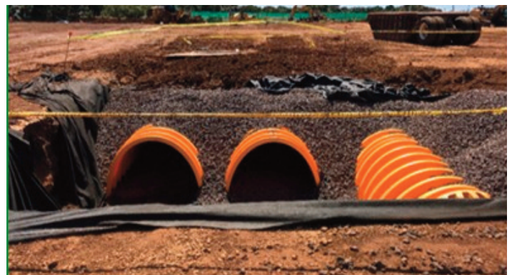
Honor Award: Installation of underground detention basin intended to capture excess storm water runoff generated by the site.
