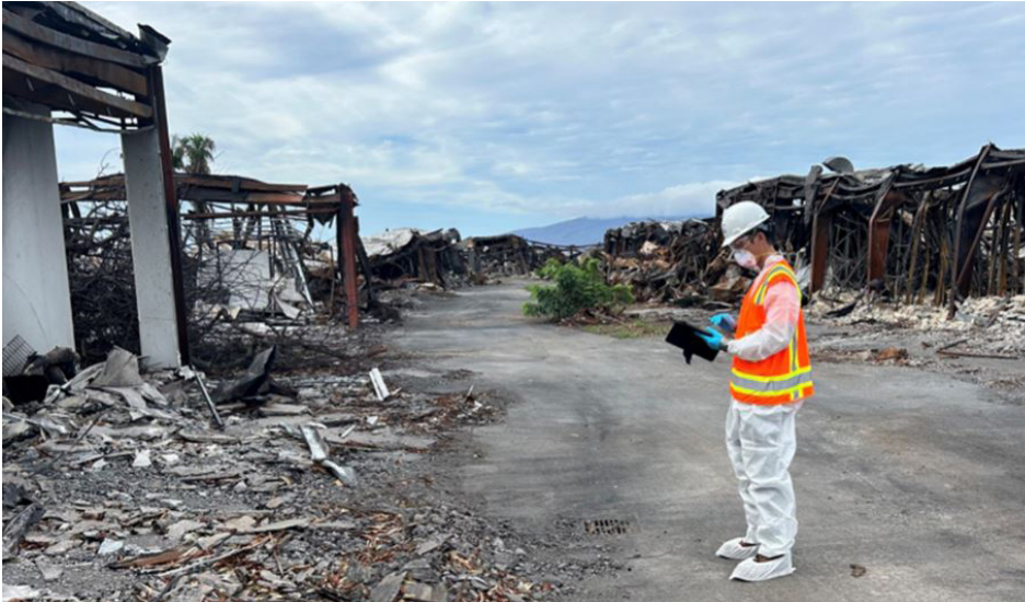
Lahaina Post-Wildfire Drainline Assessment
